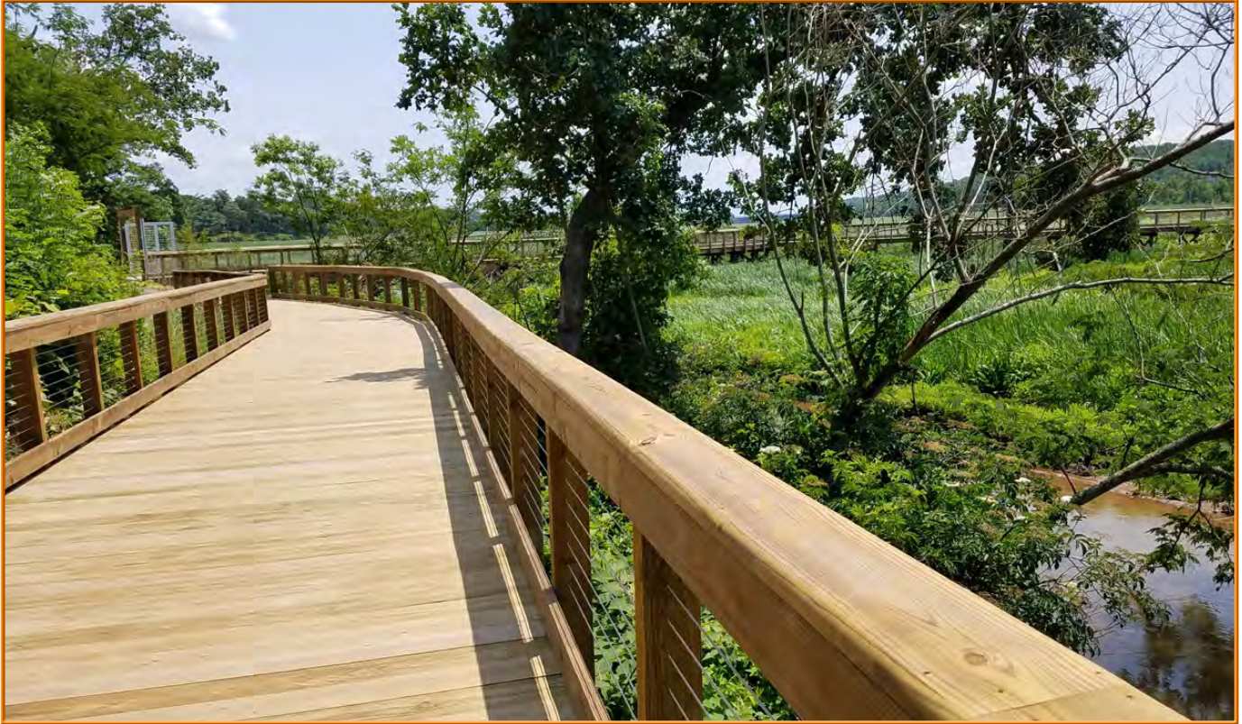
Neabsco Creek Boardwalk
