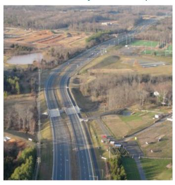
Heathcote Boulevard was designed and constructed to complete the missing section of roadway between Old Carolina Road and Route 15. RDA performed 4.7 miles of CEI and QC management to ensure the quality of the new construction.
