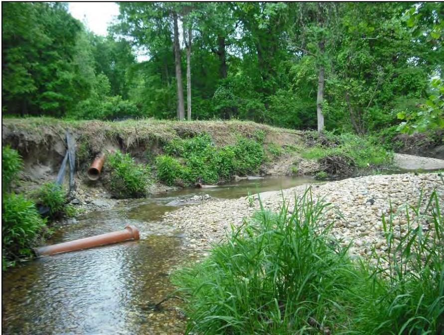
**Photo 716: Collapsed pipe on the left bank of Reach 650-A.**
