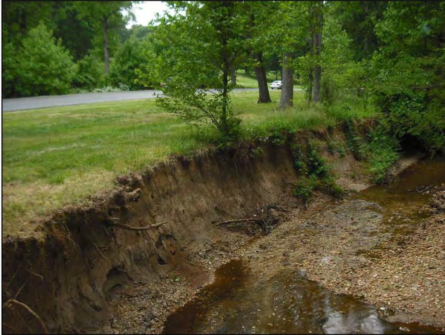
**Photo 710: Bank scouring near Fuller Road, along Reach 650-A.**
