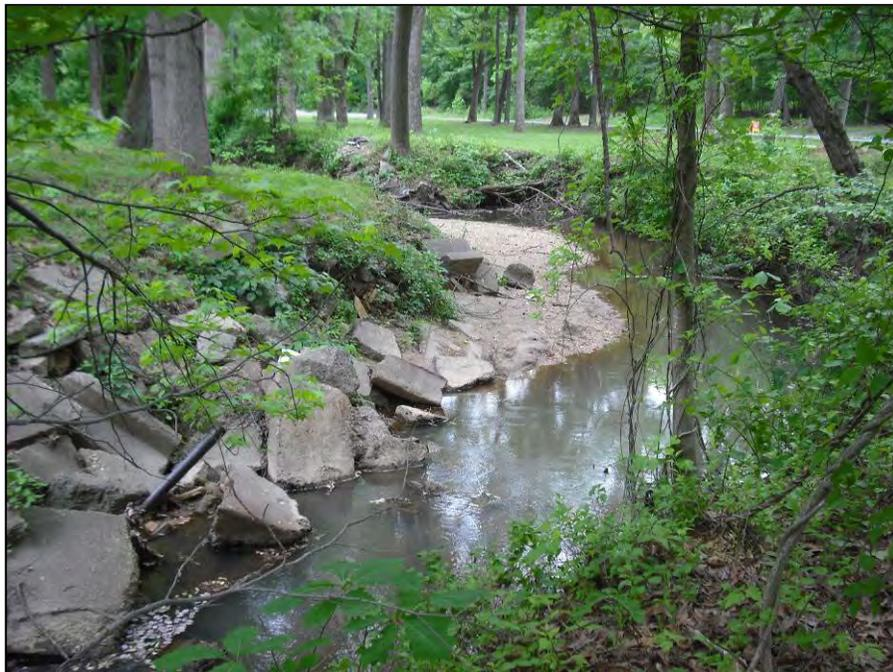
**Photo 686: Concrete rubble bank armoring in response to channel erosion along Reach 650-A.**
